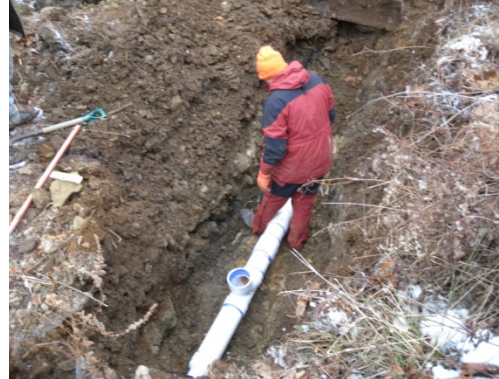
Figure 9. Air separator in trench
