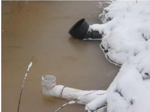
Figure 6. Tee on feeder pipe.
