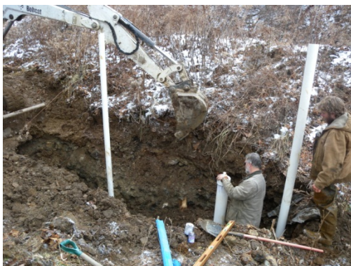
Figure 10. Inlet, outlet and air receiver.
